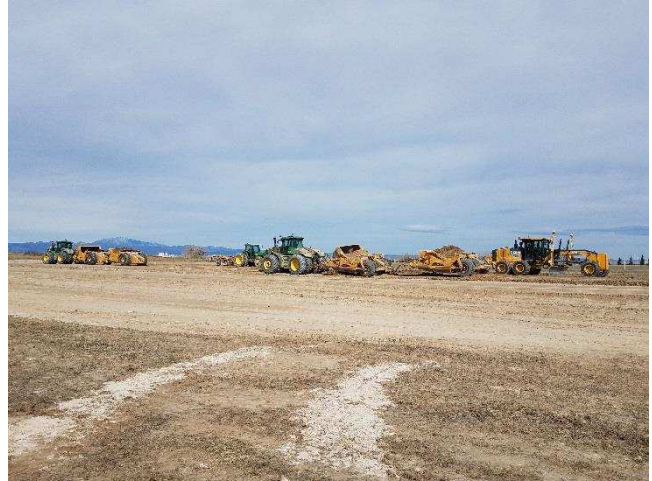
P-152 embankment fill along runway alignment.
