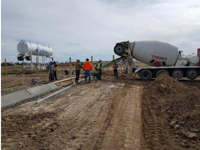
Pouring v-ditch section along irrigation system A.
