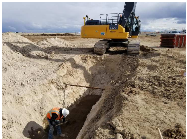
Installation of treated water line on airport property.
