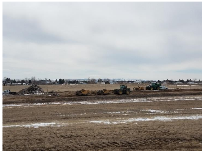
Stripping topsoil from permanent stockpile area near Contractor staging area.
