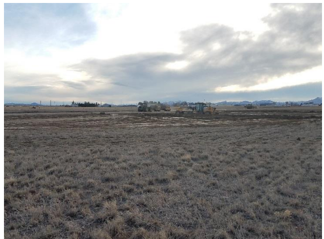
Forming Northern detention basin after topsoil removal.
