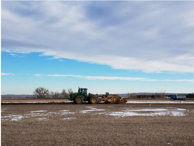
Topsoil stripping on North end of existing runway.
