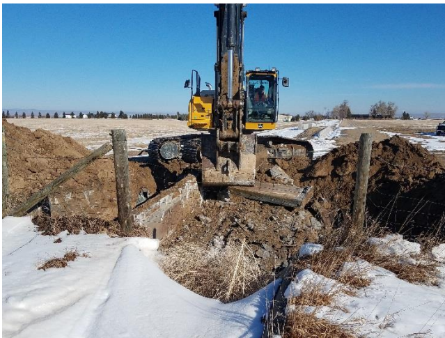
Demolish irrigation structures near irrigation system E.
