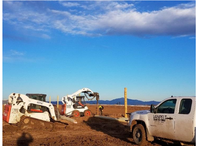
Fencing crew boring holes for brace posts.
