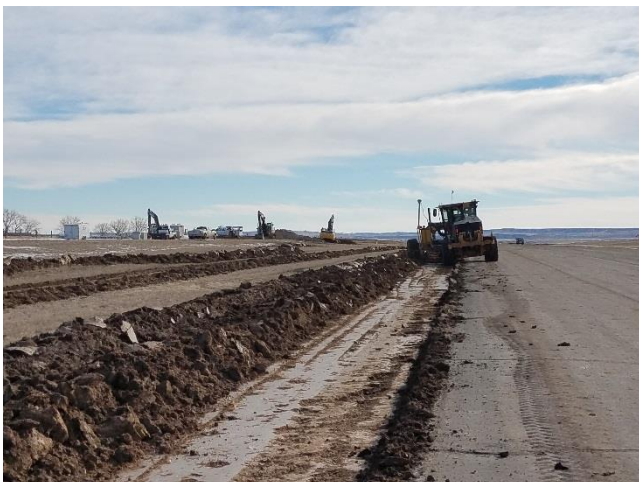
Stripping topsoil near runway on North side of existing 8/26.
